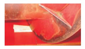
8. Wedge the panels tight against the bottom of the trough with the wooden shims supplied.
